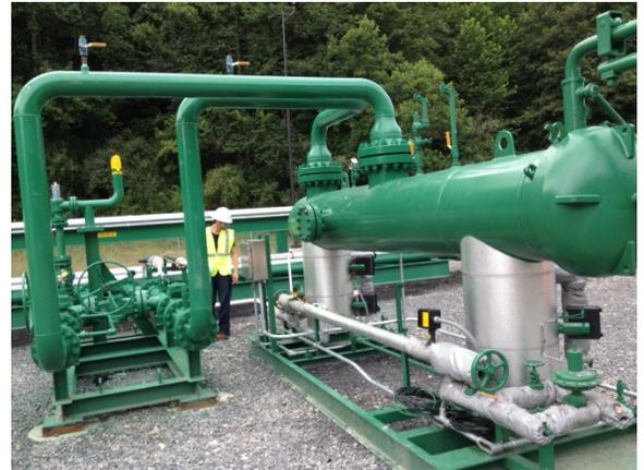
An ongoing trend has emerged toward modularization of piping and equipment onto transportable “drop-in” skids during the engineering phase of projects. As more owners and contractors realize the significant advantages and construction benefits of modular design, this trend will continue.
